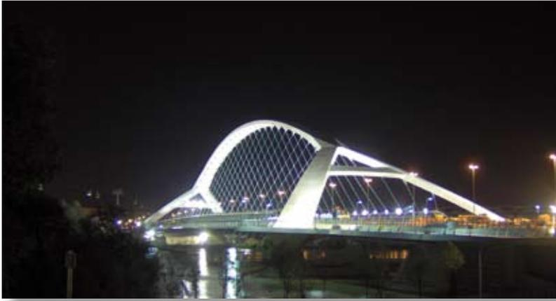
The Third Millennium Bridge is a white bowstring arch bridge. The concrete bridge has a deck width of 43 m and a main span of 216 m, making it the biggest span of this type built to date.
